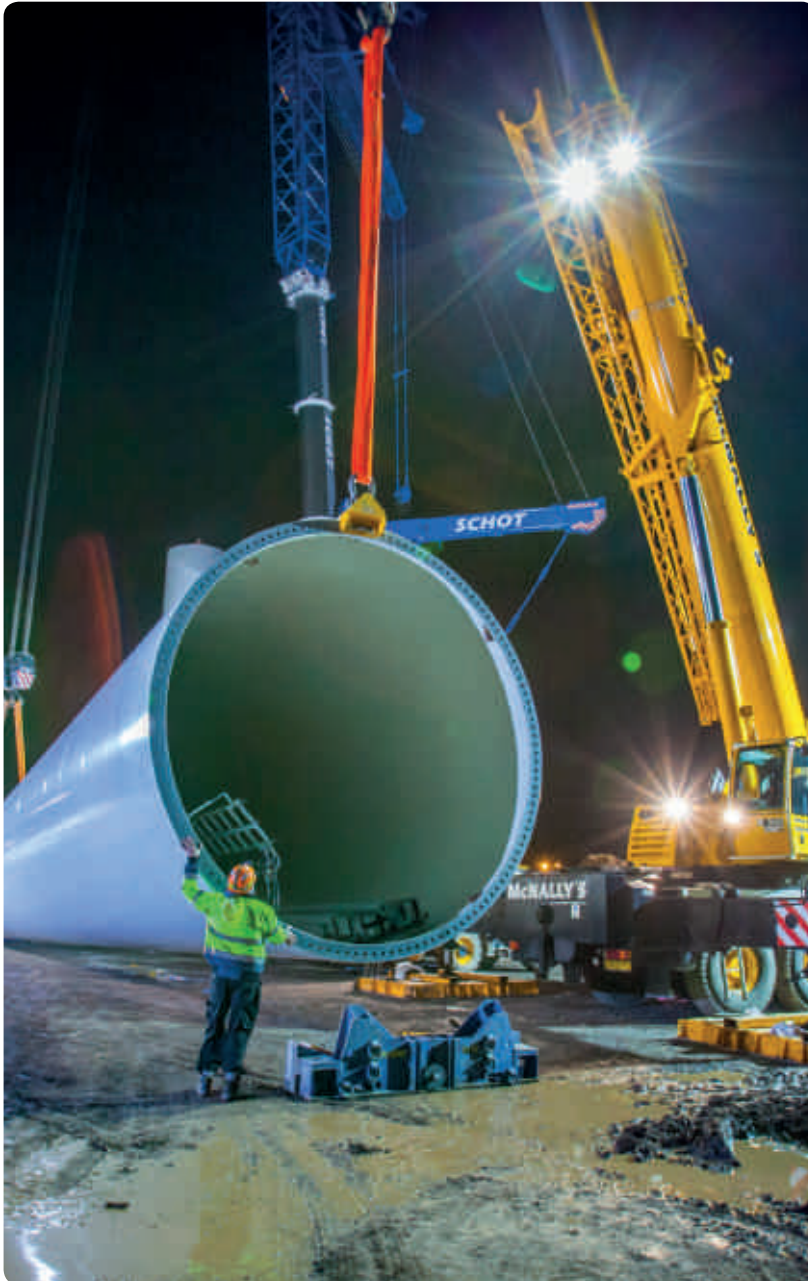
Construction of Thrive Renewables (Severn) Ltd wind farm near Bristol
